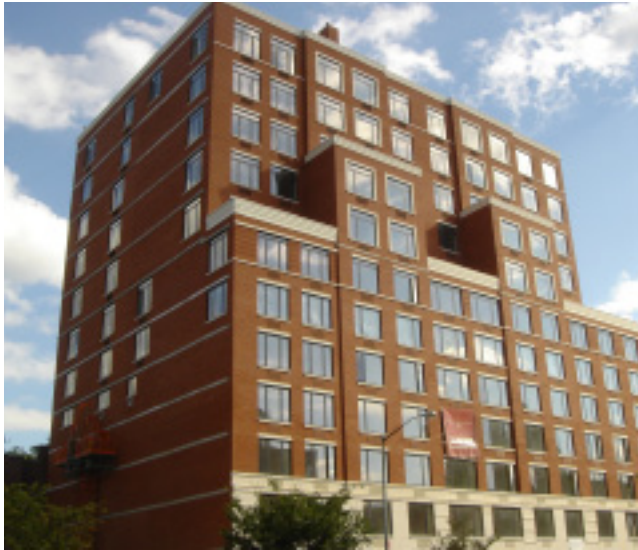
A polyester powder-coat finish from PPG Architectural Powder Coatings was applied to the aluminum windows in The Lenox, a stately residential development on Harlem's Lenox Avenue in New York. Photo courtesy Crystal Extrusion Systems
