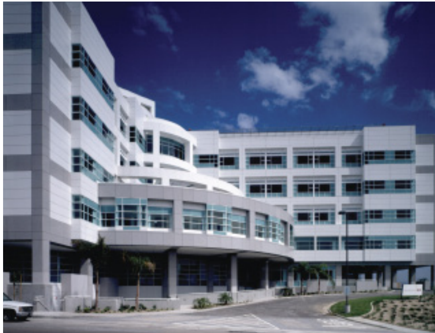
Superdurable polyester powder coatings were applied to exterior aluminum curtain-wall elements of the Mission Hospital in Mission Viejo, CA. Photo courtesy of Akzo Nobel/Interpon Powder Coatings
