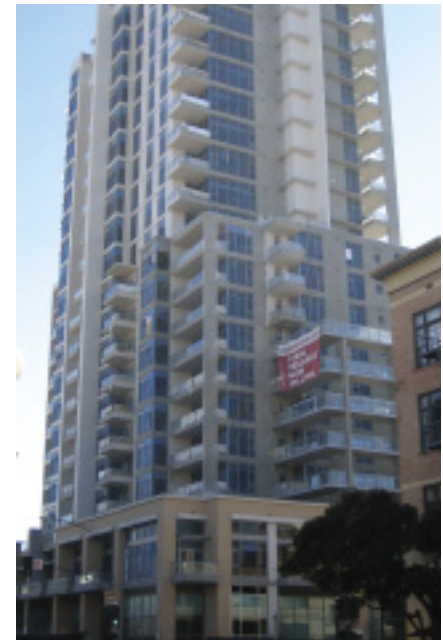
Powder coatings based on fluoropolymer resins were applied to exterior window and door extrusions of this high-rise condominium building in San Diego. Photo courtesy of Akzo Nobel/Interpon Powder Coatings
